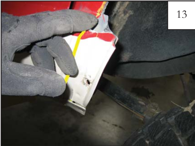
Along front fender well edge, cut through sheet metal down to the flare-out feature at the bottom.
