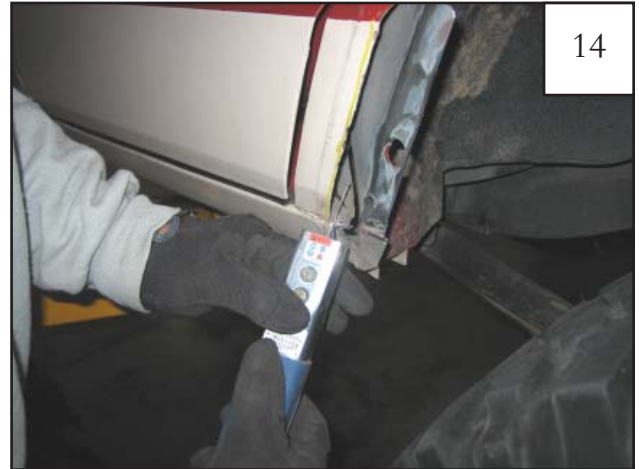
Carefully cut only the outer sheet metal layer from the flare-out feature down, leaving the inner sheet metal layer intact.
