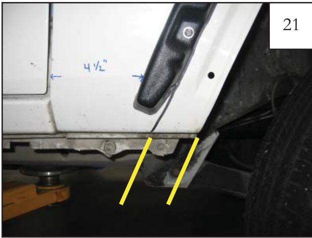
21 At end of inner pieces extend trimming line so that it is parallel with the wheel well opening instead of following inner piece curvature.
