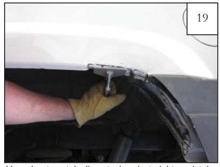
Use sheet metal pliers to bend straightened tabs back and up into wheel well.
