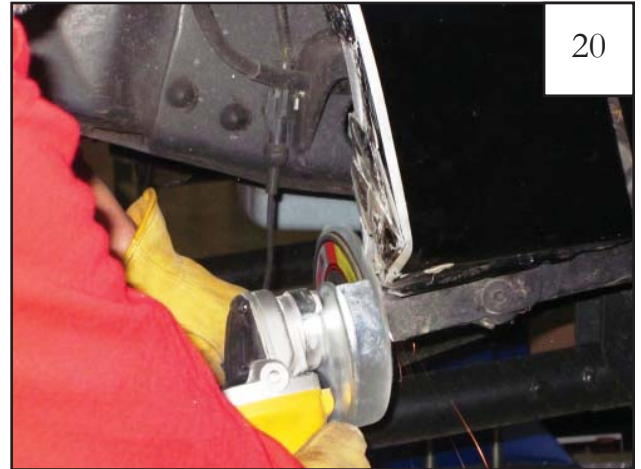
Using a hammer and an angle grinder, flatten tabs then grind down any sharp edges.
