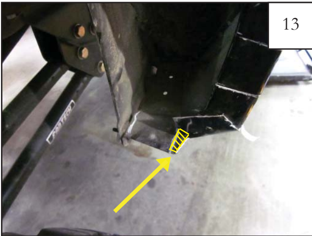
Using a Sawsall, cut off outlined area.
