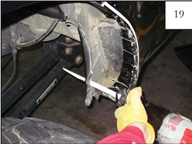
Using a Sawsall, cut along reference line.
