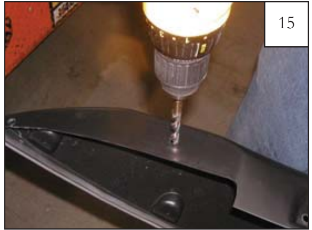
Using a 5/16" bit, drill holes at indents located at ends of Front Main Flare and Front Bumper Pieces. 2 places each part.
