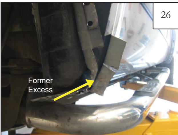
Cut off metal that overlaps outer sheet metal.
