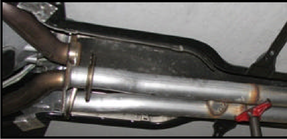
Photo 1: Factory H-Pipe Removal
